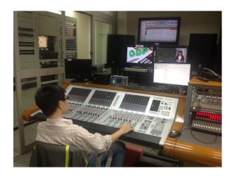
The delivery was included in Vista 1 Compact 32 Fader, Sennheiser microphone 06 pcs E 912-S BK, 2 pcs MKH 60-1, 08 pcs MKE 2-P-C, 8 sets Ew 512 G3-C, 2 sets ASA 1, 02 sets NT 1-1-EU, 02 sets A 2003-UHF, 02 sets GZG 1029, 2 sets GZP 10, 20 sets MZQ02 together with 04 pcs Genelec 8030BPM with wall-mount brackets and floor stands.
